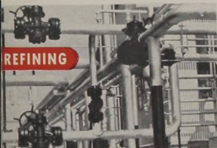
Nordstrom Gear Operated Hypresal Valves on dehydration lines.
