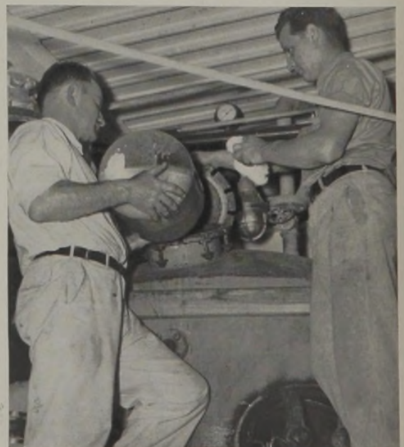
Above—A corner in Schenley Distillers Corporation's pilot plant at Lawrenceburg, Ind., showing apparatus for acetylating butylene glycol to butane diacetate, an intermediate step in converting grain to butadiene. Below left—Grain cooker in the Schenley pilot plant. Below right—Transferring bacteria to the culture tank before adding to the grain mash.
