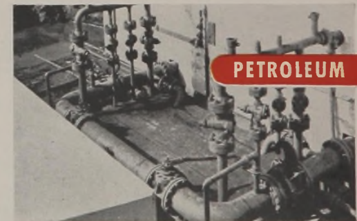
Nordstrom Valves on mud discharge manifolds and suction lines of a drilling rig.
