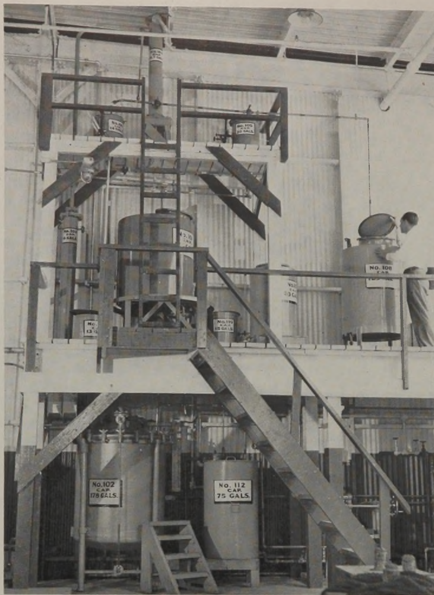
Above—A corner in Schenley Distillers Corporation's pilot plant at Lawrenceburg, Ind., showing apparatus for acetylating butylene glycol to butane diacetate, an intermediate step in converting grain to butadiene. Below left—Grain cooker in the Schenley pilot plant. Below right—Transferring bacteria to the culture tank before adding to the grain mash.
