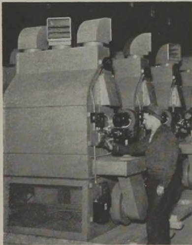
8-cylinder Cooper-Bessemer gas engine at Port Neches Butadiene plant.
