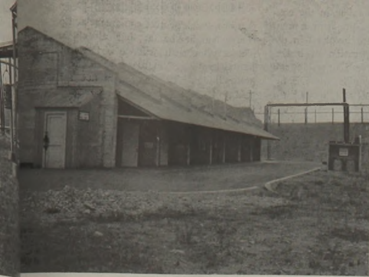
Fig. 3—Building divided into several bays by concrete fire walls. One piece of equipment is placed in each bay and scrapped process material stored in the shed at the right.
