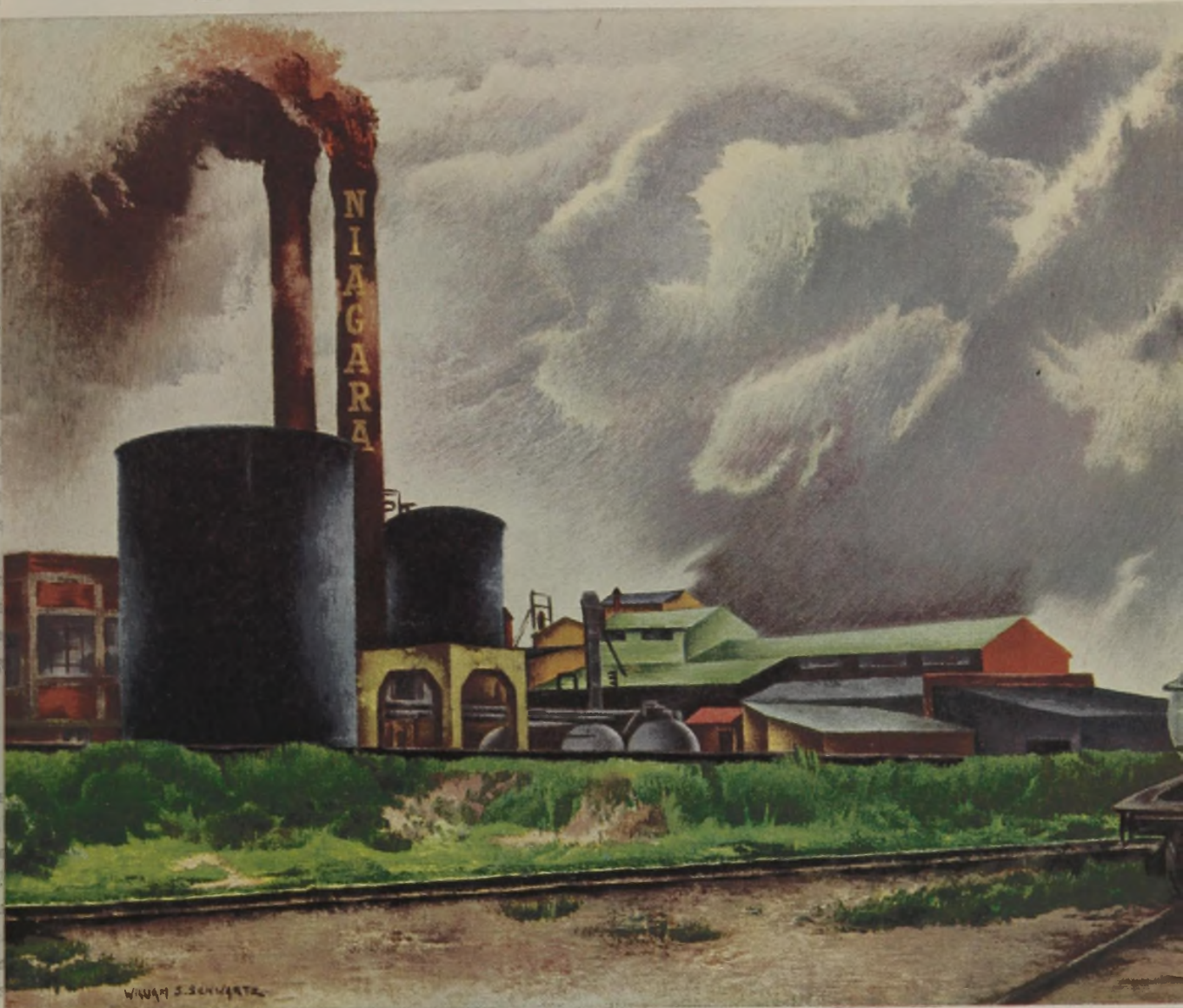
Covering an area of nearly thirty acres, Niagara Alkali Company's plant at Niagara Falls, N. Y., is one of the most modern and efficient of its kind in the world
