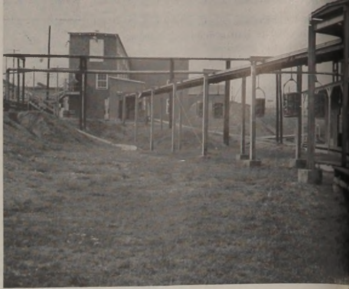
Fig. 2—Monorail system used to move a large number of relatively small amounts of water-wet, slightly flammable material between buildings. Containers spaced to prevent propagation in case of fire.
