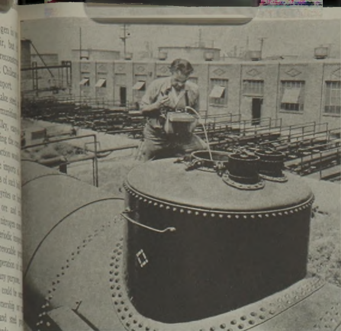
Sampling tank car air for combustible gases.
