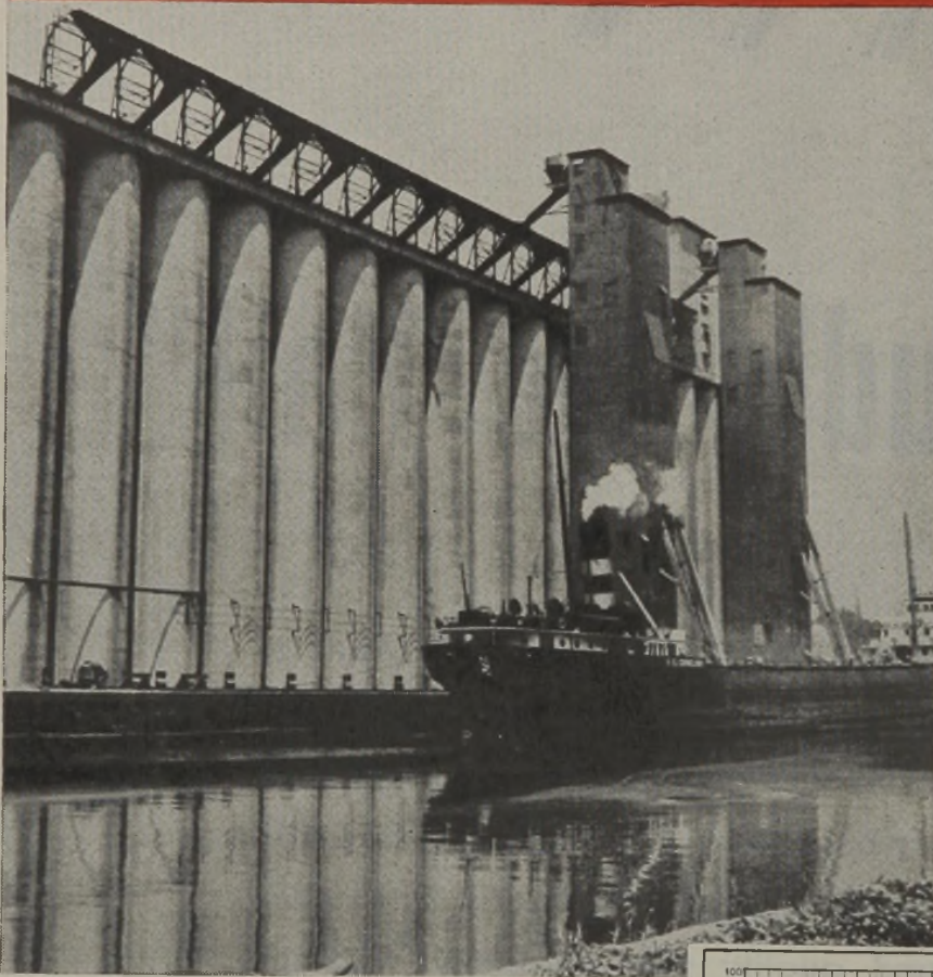
(Above) MAJOR WEAPON IN THE FIGHT against loss of stored grain and milled products due to damage by insects is Cyanamid's Liquid HCN. The effectiveness of this modern industrial fumigant is steadily saving greater quantities of food to help protect America's position as "Bread Basket of the World."
