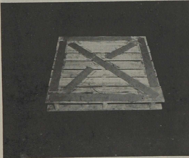
Official U. S. Navy Photos (BuS and A—NSOTC) Suggested method of placing chipboard strips on pallets
