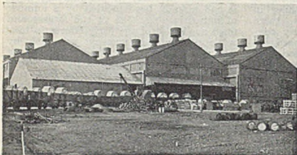
General view of the loading bays
