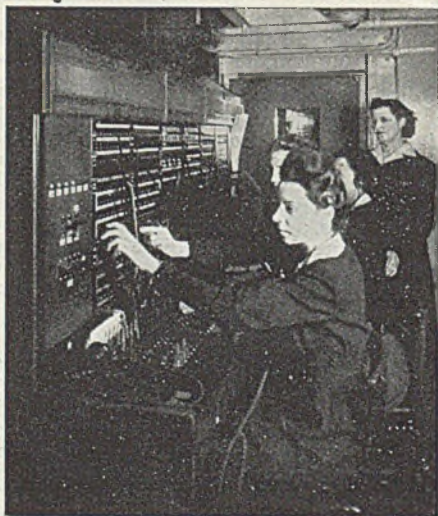
Two panels of the G.E.C. 3-position switchboard on the "Queen Elizabeth"
