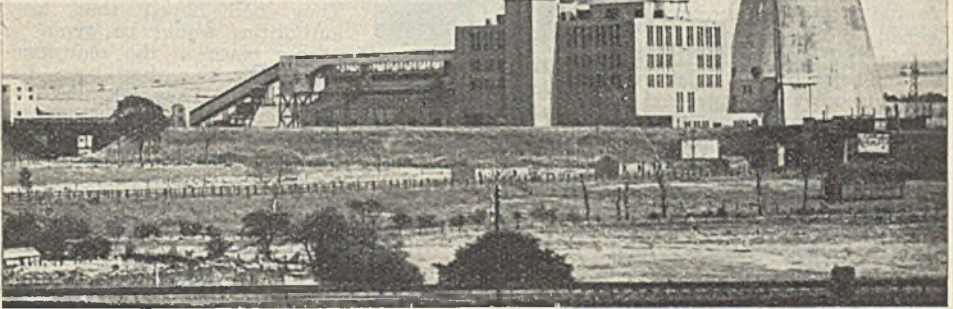
View of the Whitebirk Station of Blackburn Corporation, where last week a 70 MW extension was officially commissioned by MR. GEORGE TOMLINSON, Minister of Education
