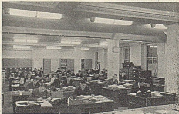
Fluorescent lighting in a West End insurance office. Philips' 80 W lamps are installed
