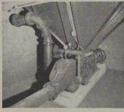
Used to convey dry pulverized materials from pulverizers, collector screws, bins, silos, hopper-bottom cars, etc. Capacities to 300 tons an hour. Convey materials as far as 3600 feet; elevation to 300 feet.
