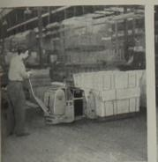
REVERSE BUTTON and guide handle eases Transporter below skid or pallet, and load is ready to be raised to moving level. Requires no skill, no muscle work—just thumb pressure.
