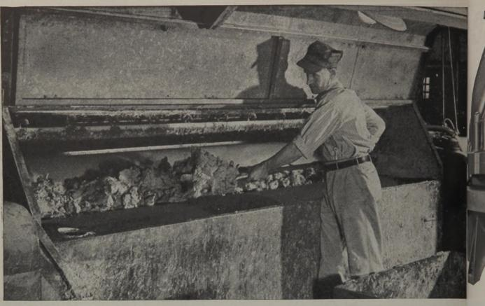
Making GABLOCK 7021 Compressed Asbestos Sheet Packing at the Garlock factory.
