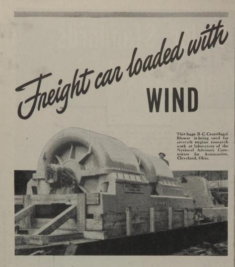
This freight car packs hurricanes! It's loaded with a Roots-Connersville Centrifugal Blower that in just one minute can push the air out of a 10' circular tunnel, 450 feet long. Or, it can blow a gentle breeze, too, if that's what is wanted.
