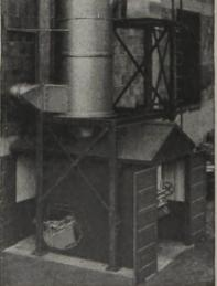
This Schneible Multi-Wash System controls a troublesome fume condition in a process plant.
