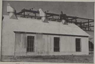
Whether it's used for a one-story utility building or a multiple-story factory, J-M Corrugated Transite meets all the modern requirements for attractive design and streamlined construction. It builds fast! And it's built to last! Corrugated Transite is a rigid asbestos sheet that provides durable, weatherproof walls and roofs for buildings of every size and design.
