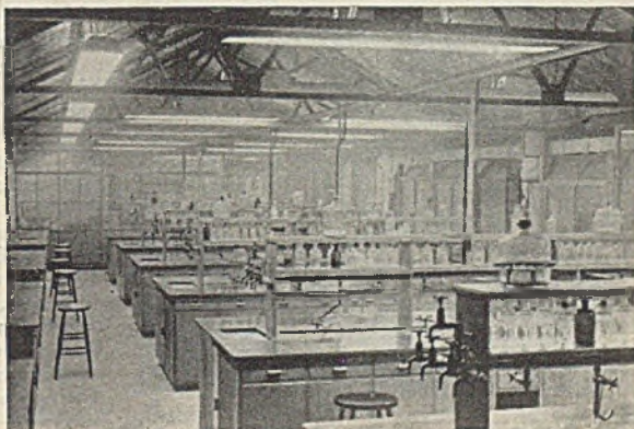
View of chemical laboratory extension, University College, Southampton, lighted with Mazda fluorescent lamps
