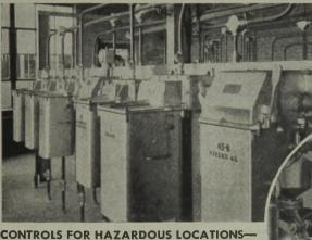
Westinghouse motor control equipment is available for all types of chemical plant applications. Photo shows group of Class 11-202 cor-rosion-resistant oil-immersed Westinghouse Linestarters for Class I, Group D hazardous service.
