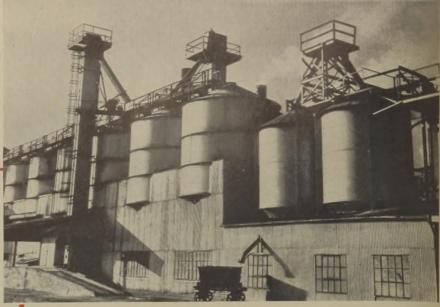
Batch house where raw materials for all fiber glass products are stored and mixed in a plant of the Owens-Corning Fiberglas Corp.
