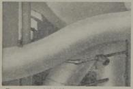
Closeup view of K & M 85% Magnesia Insulation, complete with Canvas Jacket, on portion of piping.
