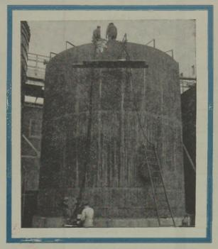
Taking SR-4 strain-gage readings during testing of field-erected vessel.
