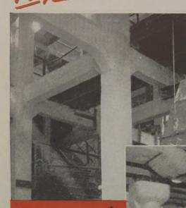
Commente salammes in muniate med plane in area next to and above furnace, where temperature is high. condensation great, and HCL. Jumes always present. Note absence of failure or disintegration of Prinfcoal-treated concrete columns after over six years of service. Formarly required painting every thirty days.
