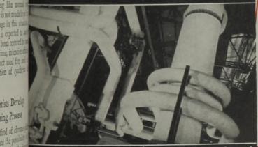
Gas and Steam Process Piping at Exit of Reformed Gas Waste Heat Boiler
