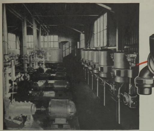
An installation of Crouse-Hinds explosion-proof CONDULETS showing the use of Type EZS Offset Sealing Condulets between Type OFC Push Button Station Condulets and Type EPC Motor Starter Condulets.
