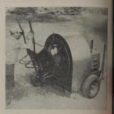
Kinetic portable revolving-drum mixer
