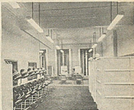
Fluorescent lighting in the ladies' salon at a Bond Street hairdressing establishment
