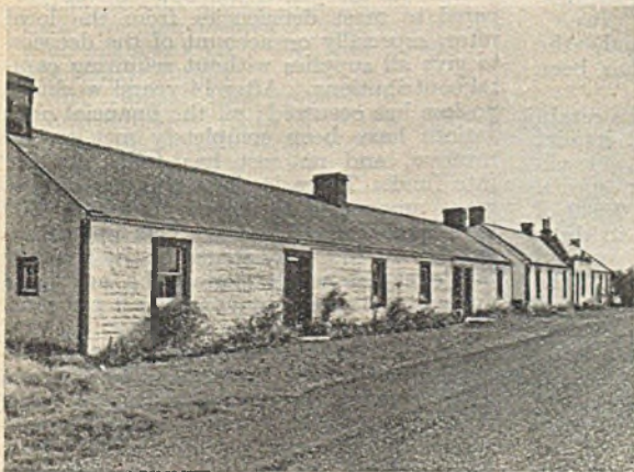
Typical under-eave distribution mains for agricultural workers cottages
