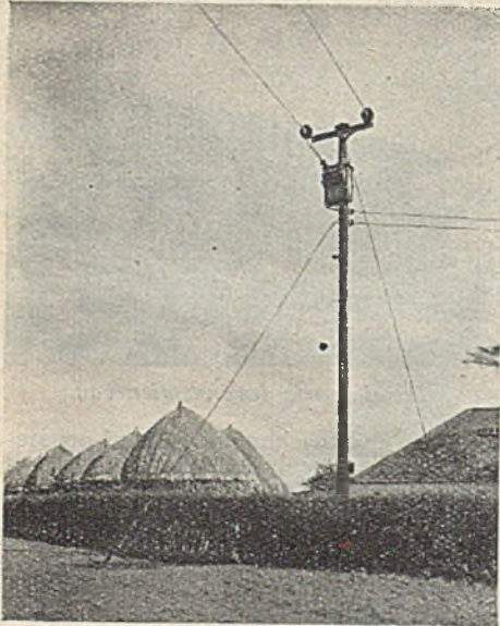
15 kVA pole-type transformer equipment for supply to farms
