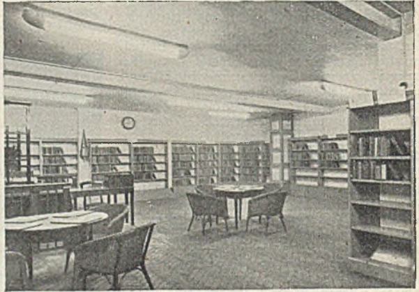
Atlas fluorescent lighting fittings with fluted Perspex diffusing covers at the Children's Library, North Kensington
