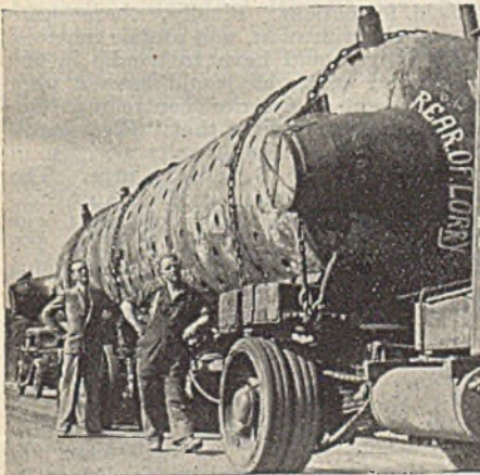
(Left) The 525 000 lb. per hr. Stirling boiler drum, towards the end of its journey to Stourport, and (right) a recent view of the station
