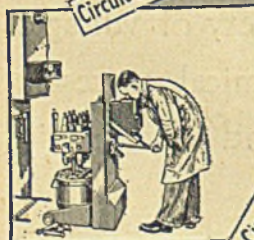
Circuit Breaker truck withdrawn from cubicle
