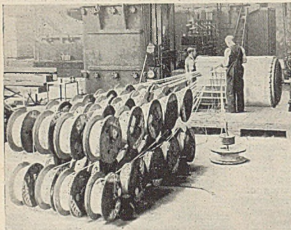
Fig. 9.—Heavy current spiral coil in course of winding
