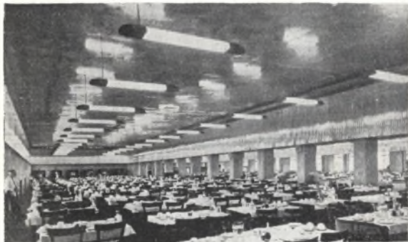
View of one half of the dining hall at Middleton Tower holiday camp, Morecambe, illuminated by fluorescent lamps in Miller-Hepworth fittings
