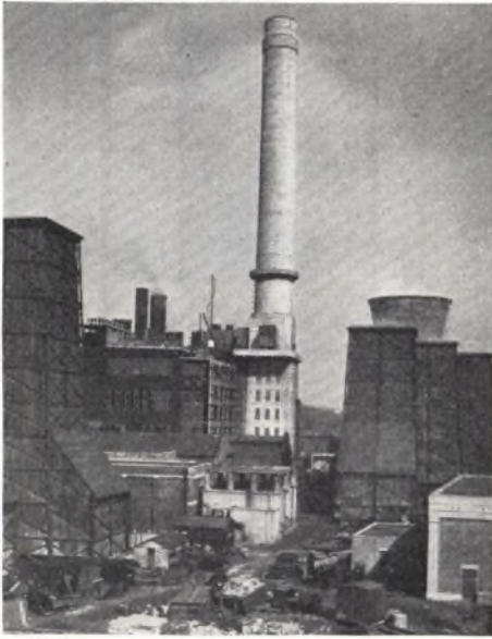
The new chimney, with the administrative block in its base. Part of the extended boiler house can also be seen
