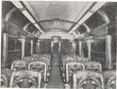
Fluorescent lighting in a Blackpool Corporation railcoach. Half saloon, looking from the centre
