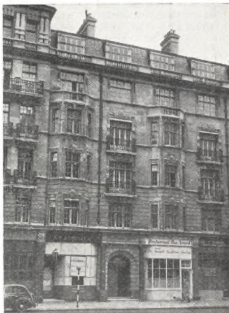
Early this week, the British Electricity Authority moved into permanent headquarters at Portland Court, 170a, Great Portland Street, London, W. The illustration above shows the entrance to the new offices
