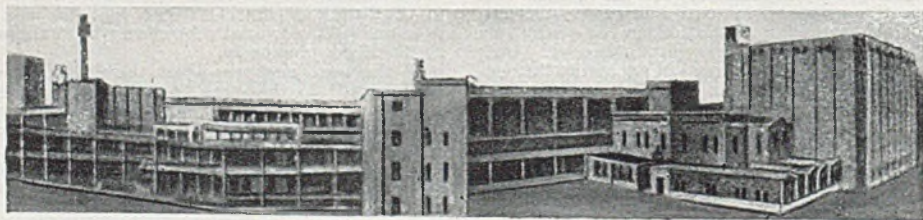
Fig. 8.—General view of the alumina plant at Arvida. Buildings at the right are devoted principally to storage and subsidiary treatment of bauxite by-products. Buildings at the left are concerned chiefly with the preparation and storage of the alumina itself.
