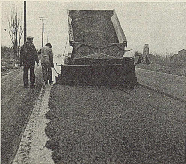
Asphalt emulsion is meeting with success in several types of road construction
