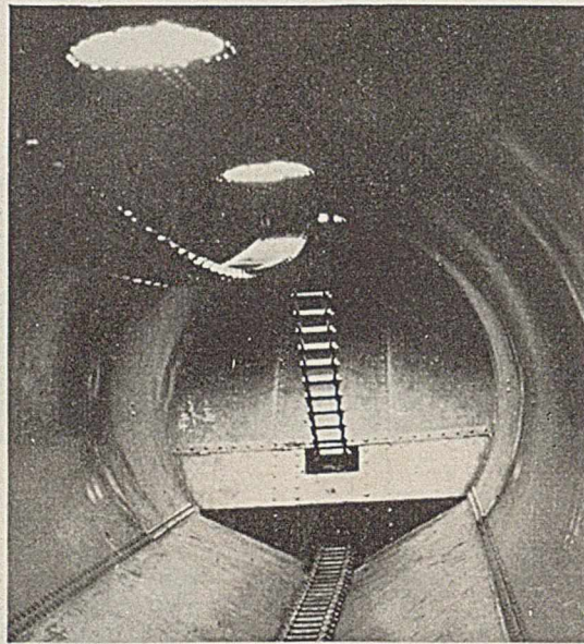
Fig. 5. Interior of Dry-Flo car, showing mechanism for unloading
