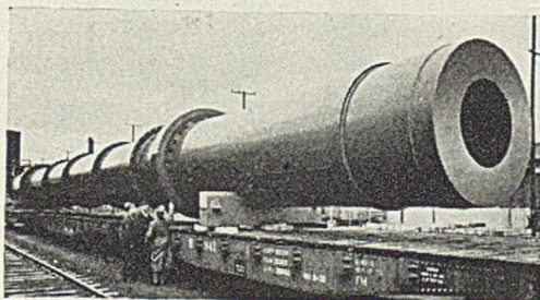
Single Kiln Three Freight Cars Long
