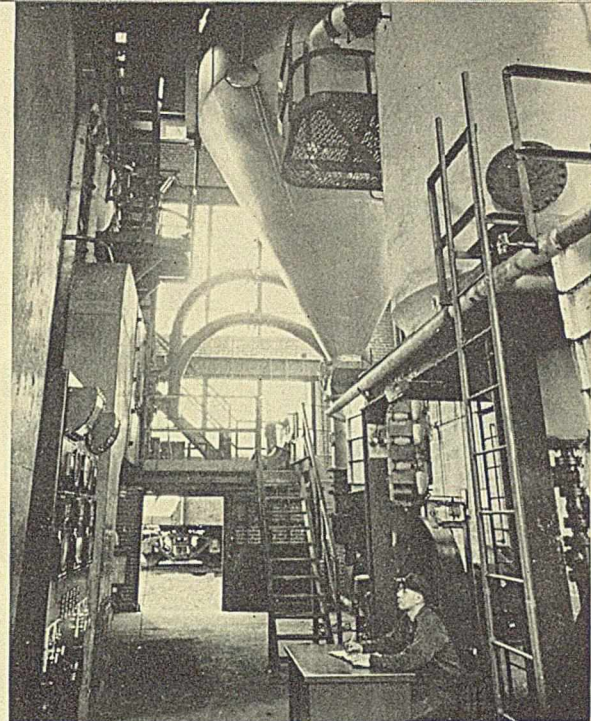
7 In this modern power plant with centralized control process steam is generated not only for the HCl vaporizers, but also for many other plant operations
