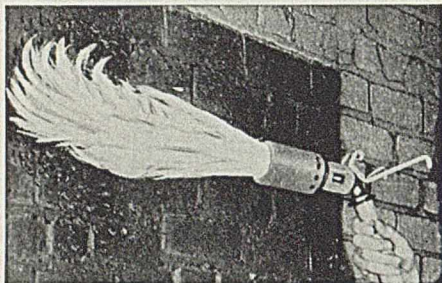
No. 5 Insto-Gas Torch with 24" flame delivers 200,000 B.T.U. Per Hour.
