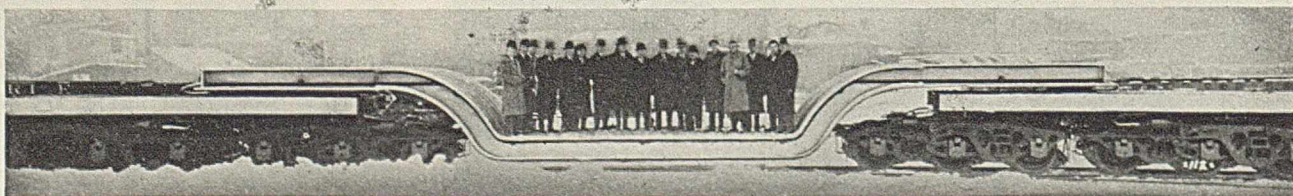
Thermit welding was used in fabricating frame of world's largest freight car
