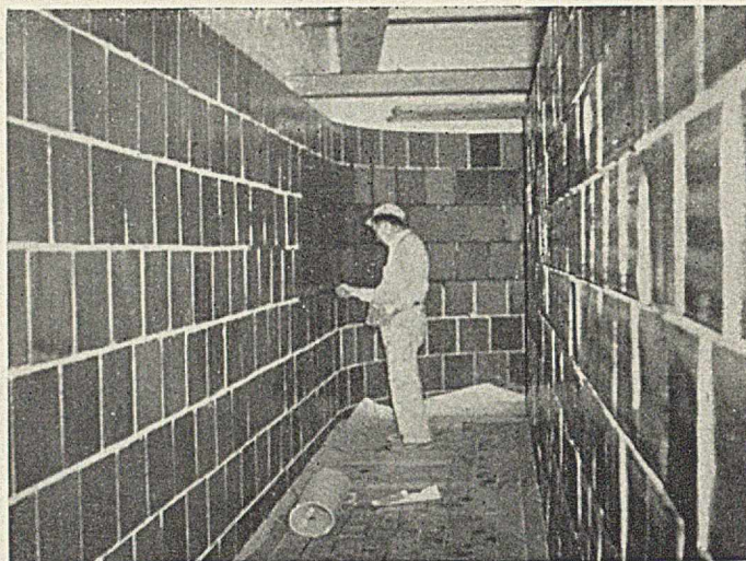
Pointing joints with Asplit resin cement in a pulp treating tank
