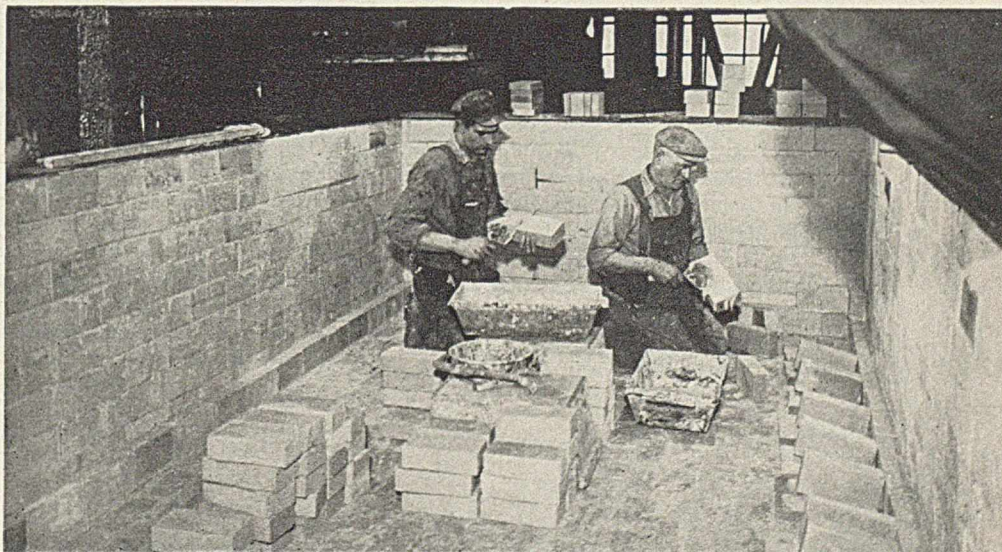
Workmen installing a two-course tank lining, using sodium silicate cement
