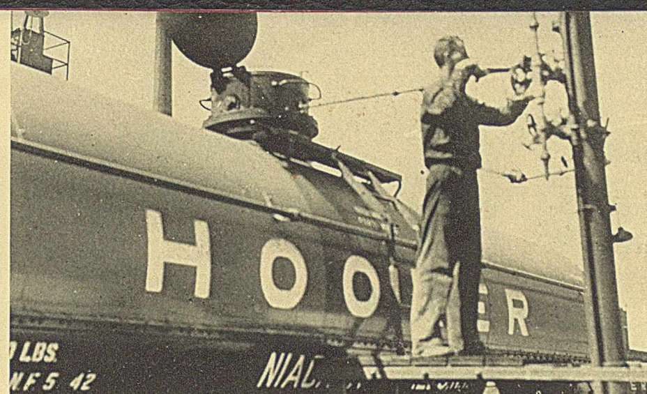
7 Liquid chlorine tank car: Liquid chlorine as required is loaded into insulated tank cars for shipment to all parts of the country
