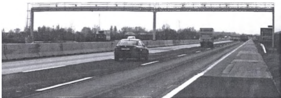
Fig.4. The example of a „Multilane Free-flow” portal
