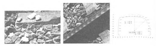
Fig.1. Typical track damages due to bad rolling conditions
