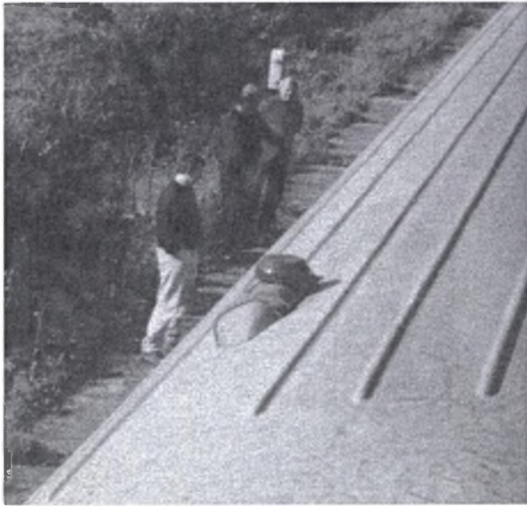
Fig.4. Installation of the IAT-Terminal in a newly designed PESA-sleeping car (PKP), the antenna is visible on the roof of the vehicle
