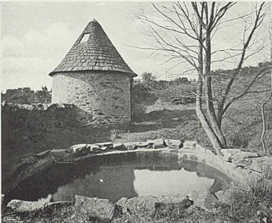
FIG. 232.—BATHING POOL AT STONEYWELL COTTAGE.
