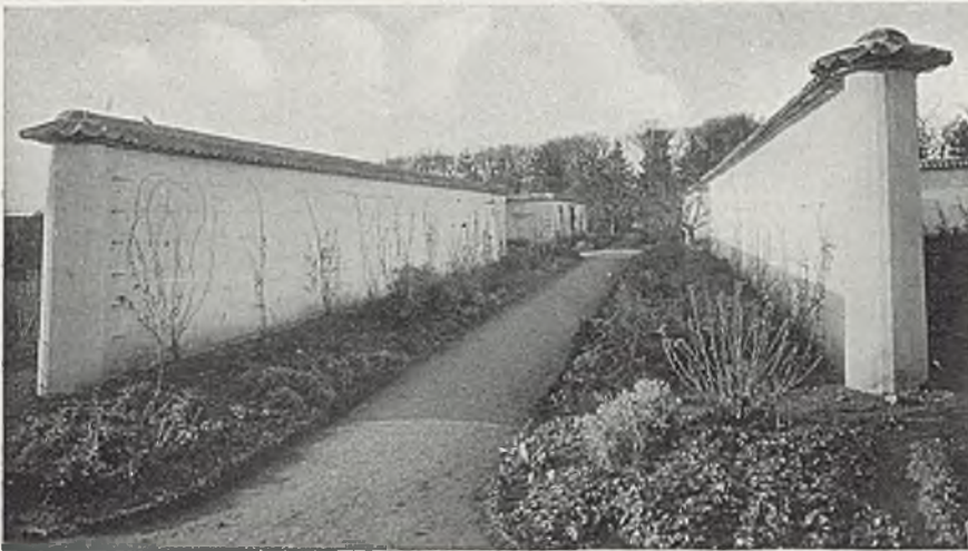
FIG. 145.—CONCRETE WALLS AT LAMBAY.
