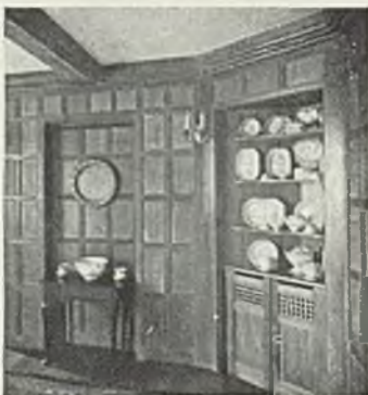
CHINA SHELVES AND RADIATOR CUPBOARD.
