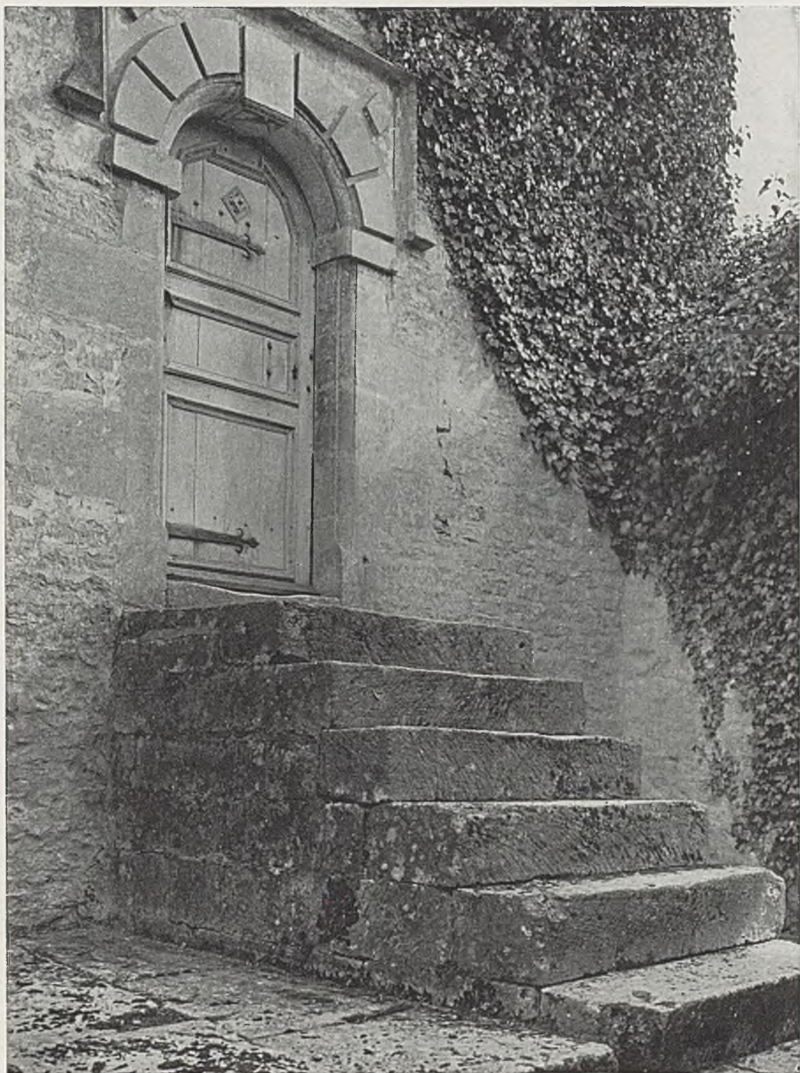
FIG. 114.—AN UNRAILED STAIR.
