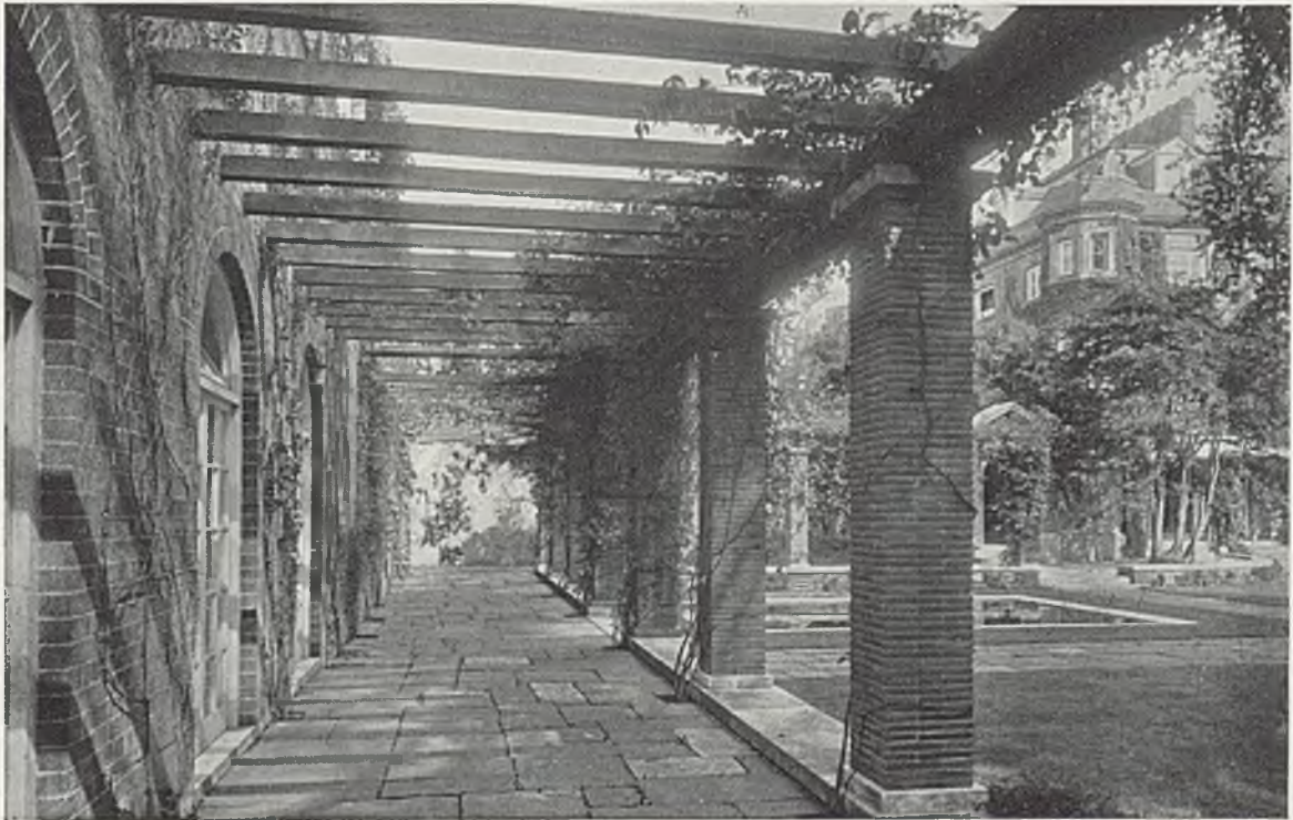
FIG. 260.—A WELL-BUILT PERGOLA ADJOINING RACQUET COURT AT ST. CLERE.
