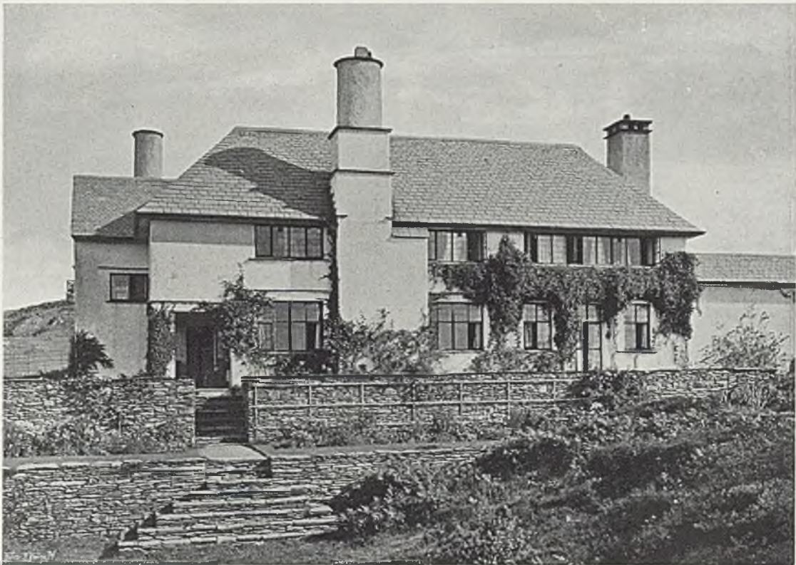
FIG. 155.—THIN SLATE STONES LAID LEVEL.
