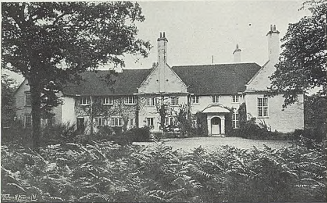
FIG. 15.—HIGH COXLEASE: ENTRANCE FRONT.
