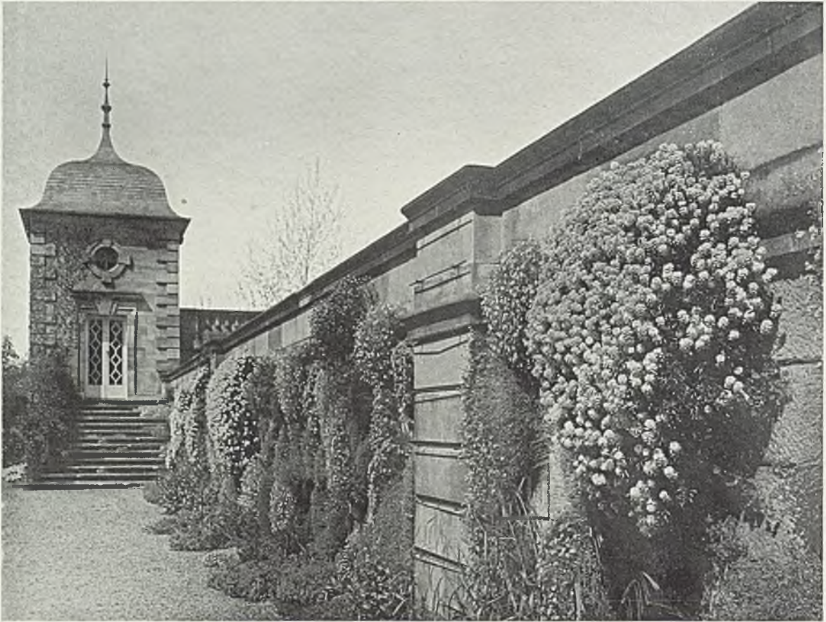
FIG. 317.—A TYPICAL SCOTTISH GARDEN PAVILION.
