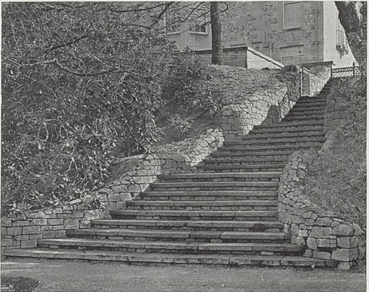
FIG. 112.—WIDENING STAIRWAY AT ARDKINGLAS.
