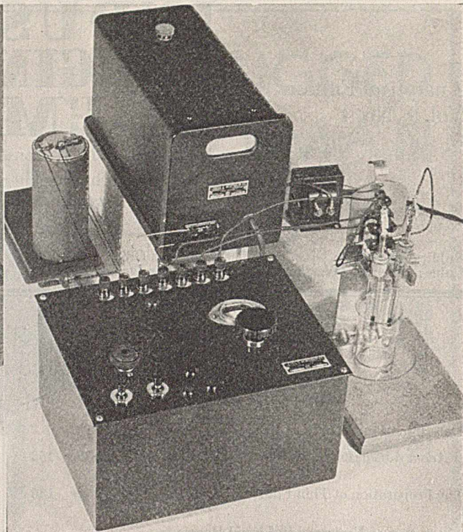
Glass Electrode with No. 7652 Guarded Potentiometer and Dual Galvanometer
