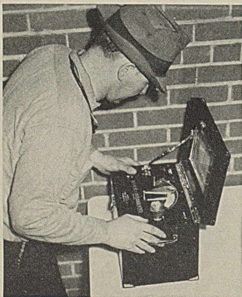
FIGURE 178. PLANT USE OF CARBANALYZER FOR DETERMINING CARBON IN STEEL
