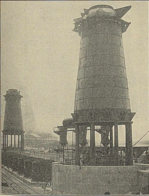
Fig. 8.—Blast furnaces under construction
