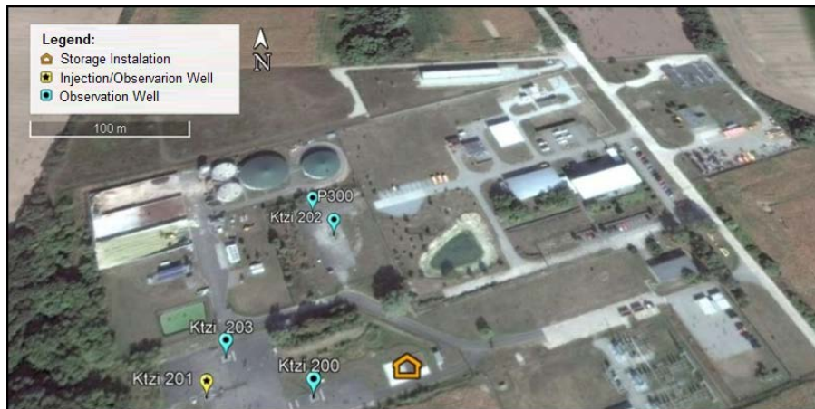
Fig. 1. Geographic location and aerial view of Ketzin site and its facilities.
