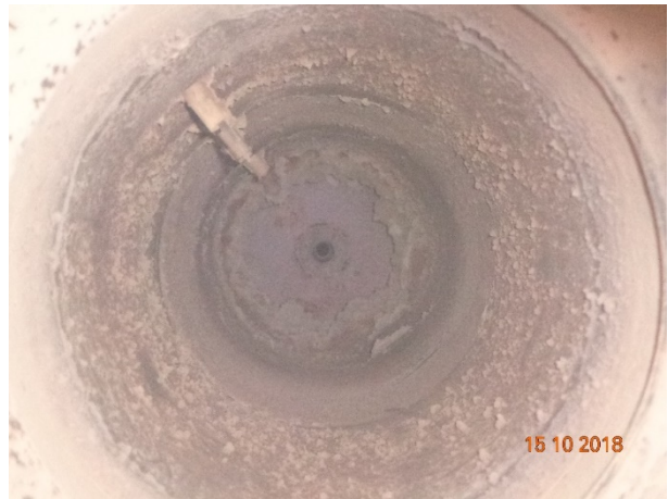
Fig.3.6. Photo of reactor interior (inner diameter 300 mm) after biomass depositions experiments. Visible thick deposit coating in upper part of reactor, close to burner (deposit thickness can be around 50-100 mm).
