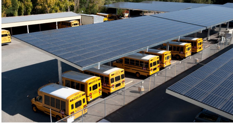
Fig. 3.1. Solar Panels Used to Offset School Energy Costs [12]
