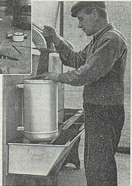
Insulating a storage heater with burnt granulated cork
