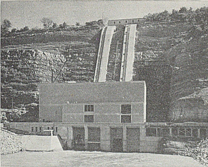
The DeCew Falls plant of the Ontario Hydro-Electric Power Commission, near St. Catharines, Ontario, was placed in operation last year. It generates 70,000 h.p. at 25 cycles. It was started in the autumn of 1945 and cost about $8 million
