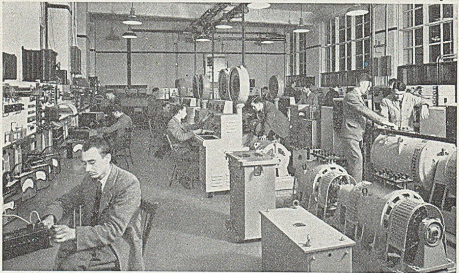
General view of the Lenz Laboratories, Stafford
