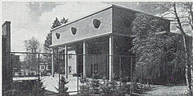
Test cells at the Arnhem testing station with 30ft head room, each equipped with a 5-ton crane, and outdoor test yard in foreground
