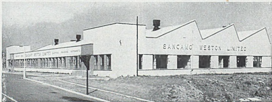
The factory of Sangamo Weston, Ltd., officially opened last week at Port Glasgow
