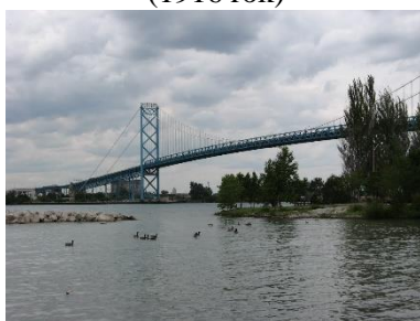
Ambassador Bridge w Detroit (1929 rok)
