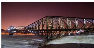
Quebec Bridge (1917 rok)
