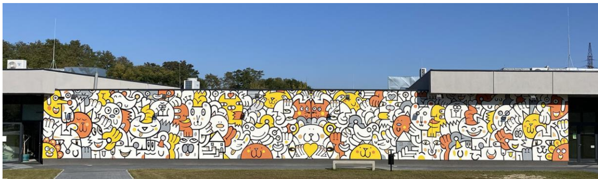
Fig. 1. The facade of the Animal Shelter, Kobylepole street in Poznań Source: K. Słuchocka
