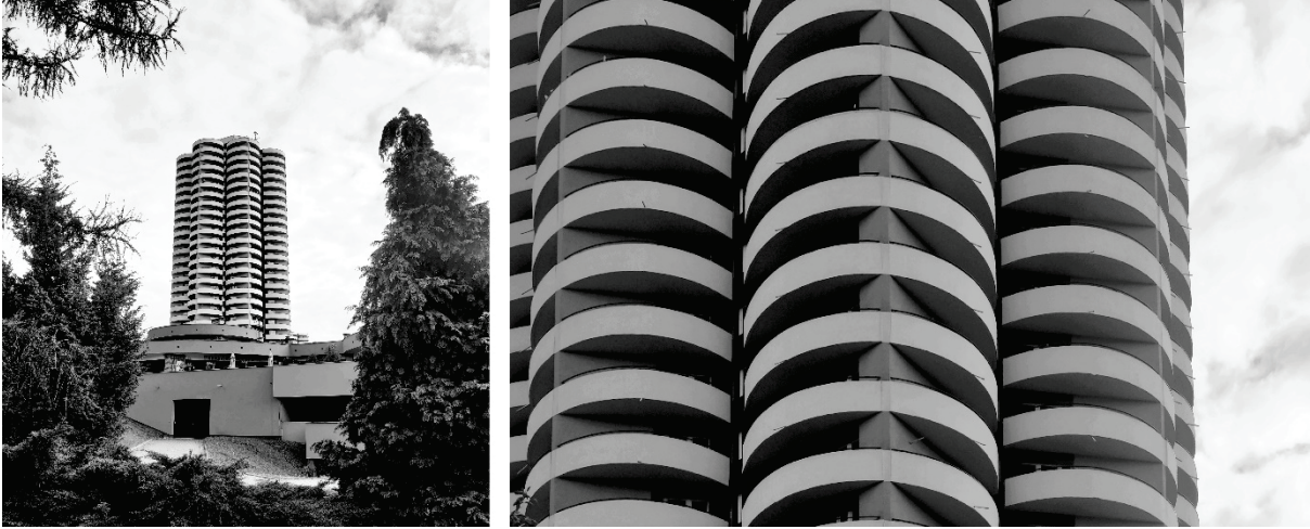
Fig. 5. Multi-family residential building commonly referred to as Kukurydza, Katowice Source: photographs by the author, 2021
