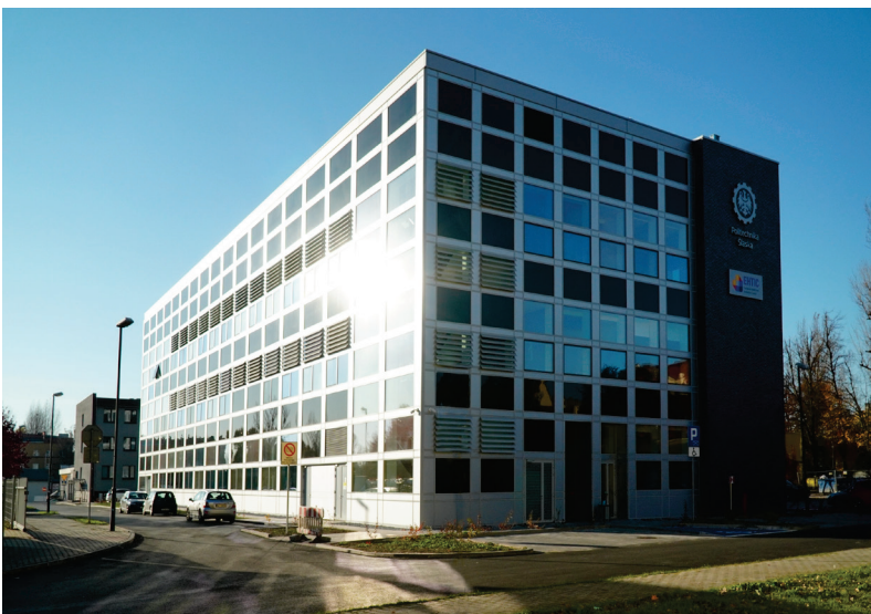
Fig. 20. EHTIC – a south-east vista, road access and technical staff entrance, September 2021. Photo by G. Wagner
