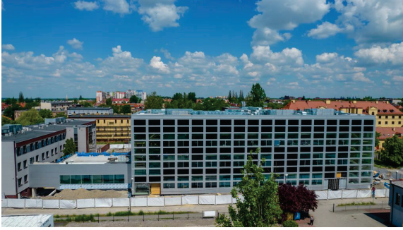
Fig. 16. EHTIC – a bird’s eye view. South façade and the building of the Faculty of Biomedical Engineering (on the left side). State of works as of 1 July 2021 (archives of the construction process)
