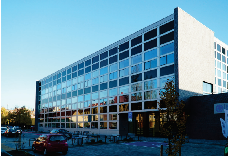
Fig. 18. EHTIC – a north-west vista, a view of the entrance square, September 2021. Photo by Grzegorz Wagner
