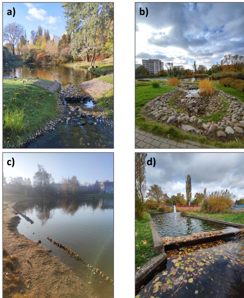
Fig. 3. Environmentally friendly solutions for water regulation: a) stone sill (Park im. Edwarda Szymańskiego in Warsaw), b) stone sills cascade (Park im. Edwarda Szymańskiego in Warsaw), c) wooden Palisade (Park Arcadia in Warsaw), d) wooden sill (Park im. Edwarda Szymańskiego in Warsaw)
