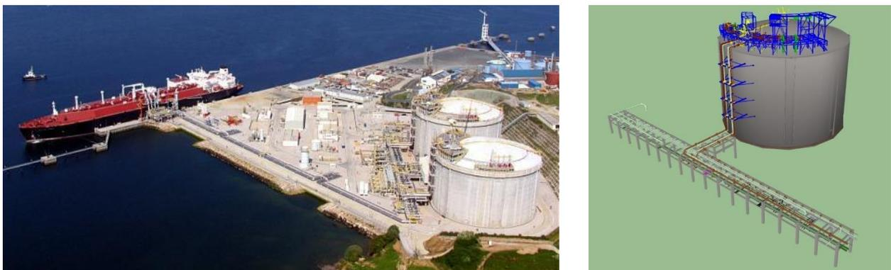
FIGURE 21: LNG PLANT USED AS CASE STUDY FOR [26] (LEFT) AND 3D MODEL OF THE STORAGE TANK, SUPPORT STRUCTURE AND PIPING SYSTEM (RIGHT)
