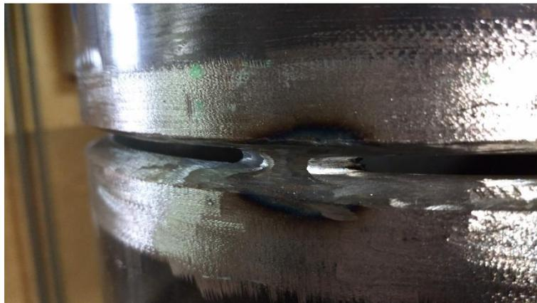
FIGURE 40: BEVELLING OF THE PIPES BEFORE WELDING PROCESS
