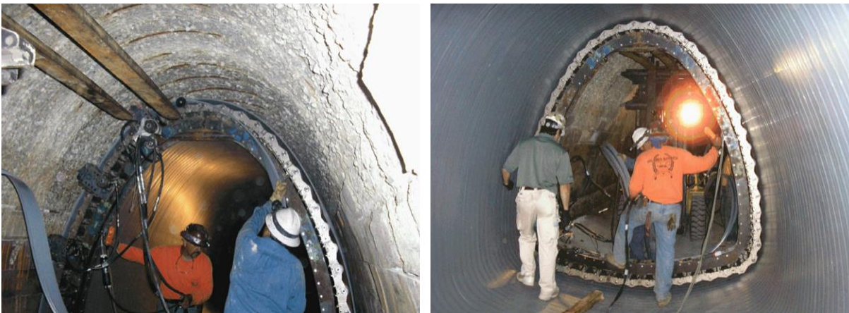
Fig.2.4.2: Sewage pipeline during and after rehabilitation [230].
