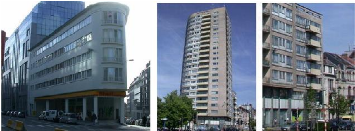
Fig.2.2.2: Structures in Brussels made partly of Purdocement [123].
