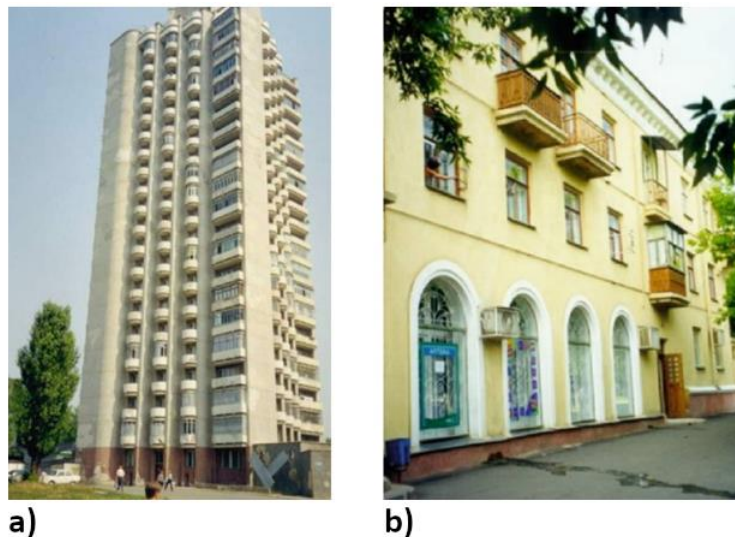
Fig.2.2.3: a) 24-storey building made of alkali activated slag-based material in Lipetsk (Russia, 1994), b) Residential building build with alkali hydroxide-activated slag-based precast elements in Mariupol (Ukraine, 1960) [62].
