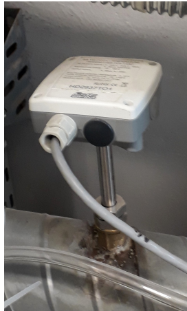
FIGURE 3.4: Air speed and temperature transducer mounted in air inlet pipe in EM mill installation
