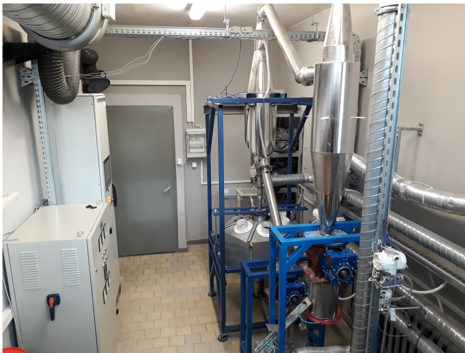
FIGURE 1.4: Dry grinding system with electromagnetic mill built at the Silesian University of Technology. Rear right — EM mill and precise classifier, front right — cyclone and transport air pipes, rear left — control cabinet for automatic control systems, front left — power supply and control cabinet for EM mill's inductor.
