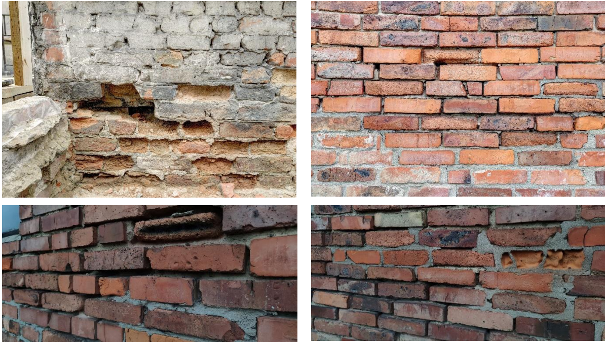
Rys. 5. Stan zachowania cegieł i spoin Fig. 5. State of preservation of bricks and joints
